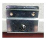
3. Install the included self-tapping screws using a cordless driver.
